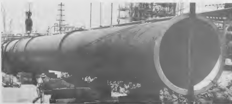
THE RING of holes at the stack's base was first positioned on the bolts on the east side and then skillfully slipped over the others. Below, the giant just she left her horizontal resting place.
